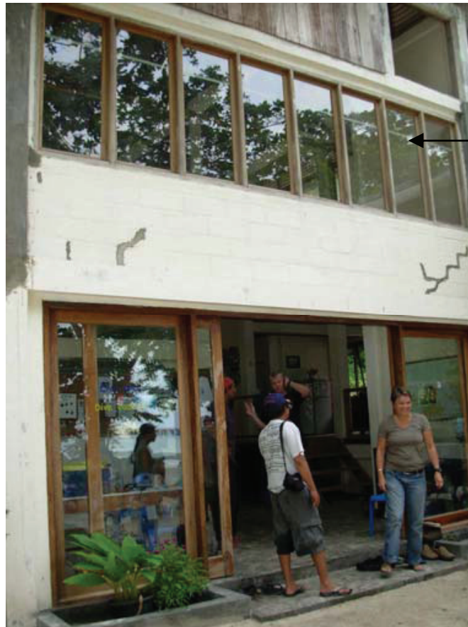
Figure 11. Lumba Lumba dive shop on Pulau Weh; arrow indicates maximum height of wave action (~5 m above sea level) on December 26, 2004.
